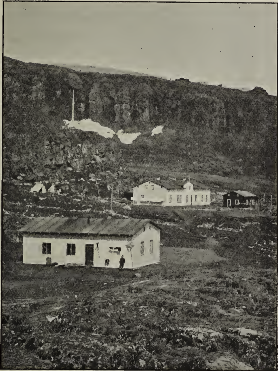
Fig. 1. The Arctic Station with the respiration chamber in course of construction.
